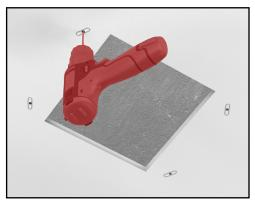
3. Drill four, quarter inch (6.35mm) holes in the center of the slotted markings. The holes must be centered to allow for fine tuning of the fixture bracket once installed.
