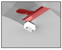
15. Apply the subsequent coat of plaster to level out the board with the existing drywall finish.
